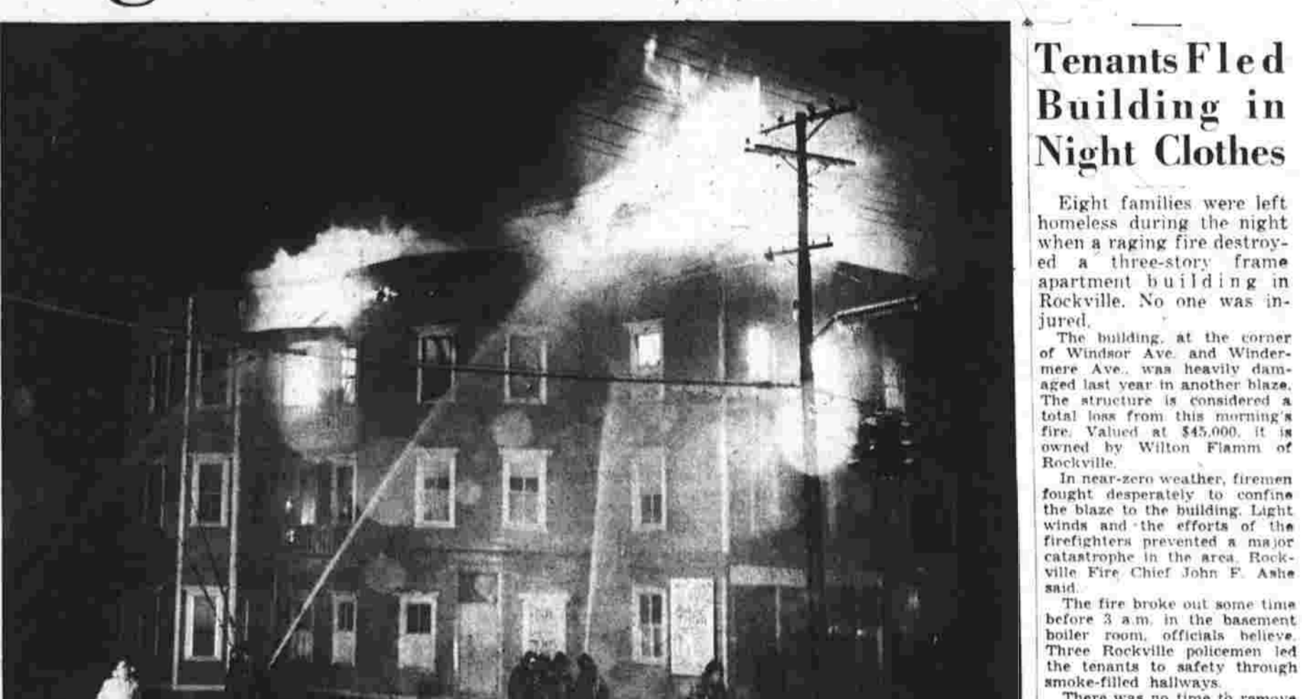
Flames break through the roof of the Flamm building in Rockville today. (Herald photo by Saterini.)
